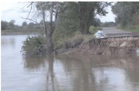
Dike breach near the village of Kępa Gostecka, August, 3 d , 2001
