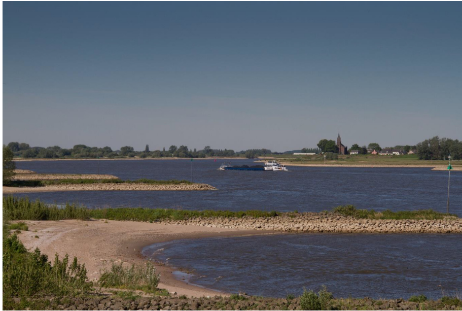
Fig. 1. The river Waal landscape with traditional groyne structures and the formation of beaches in the low-lying floodplains. (Source: https://beeldbank.rws.nl , Rijkswaterstaat).
